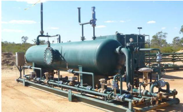
Figure 2. Separator on Arrowsmith location
